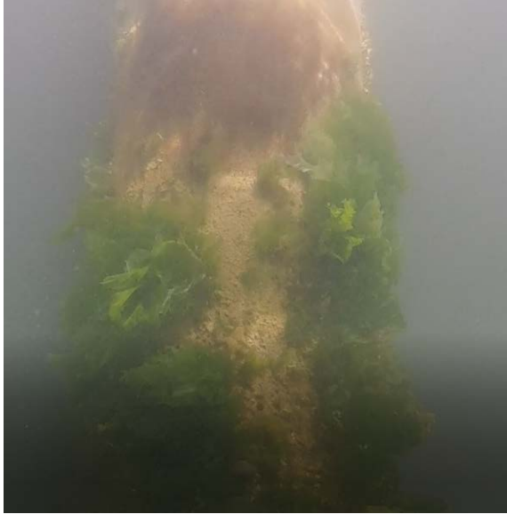
2-Typical Good (Pile D10)
