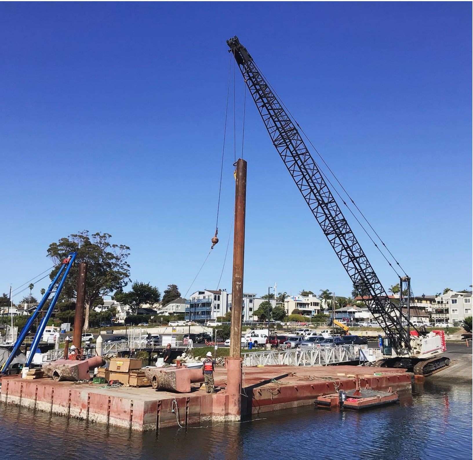
Figure 8-4: Aldo's Seawall Project
