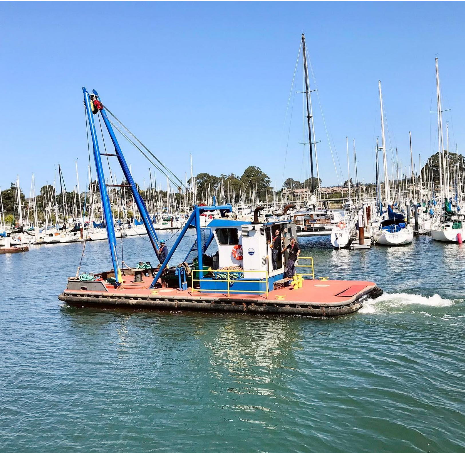
Figure 8-6: SCPD Dredging Operations.
